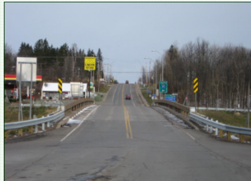
Limited space for trail on Skyline Pkwy/Boundary Ave to cross over I-35 bridge
