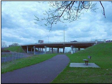
Building trail connections between East 2nd Street and the Osaugie Trail spur at 26th Avenue E would provide non-motorized users the protection of a grade-separated crossing.
